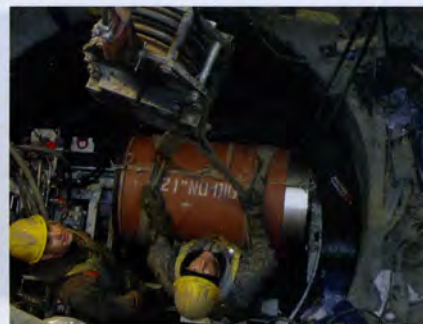
21-inch PTMT project, Edmonton, AB
